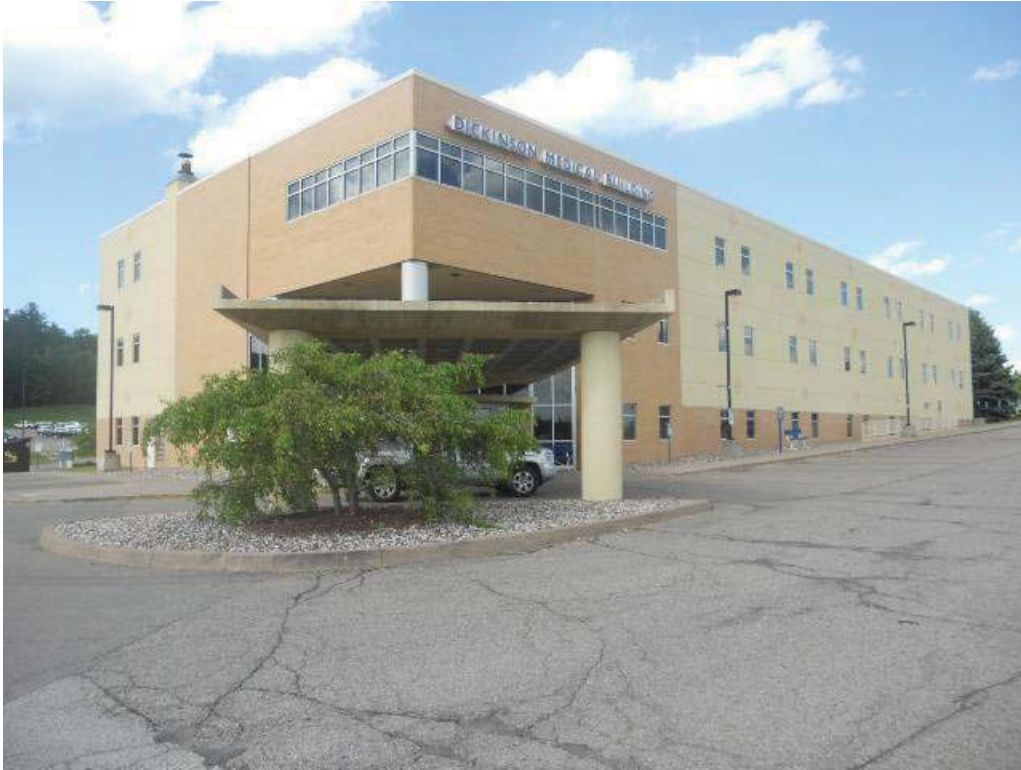
South Side of Building
