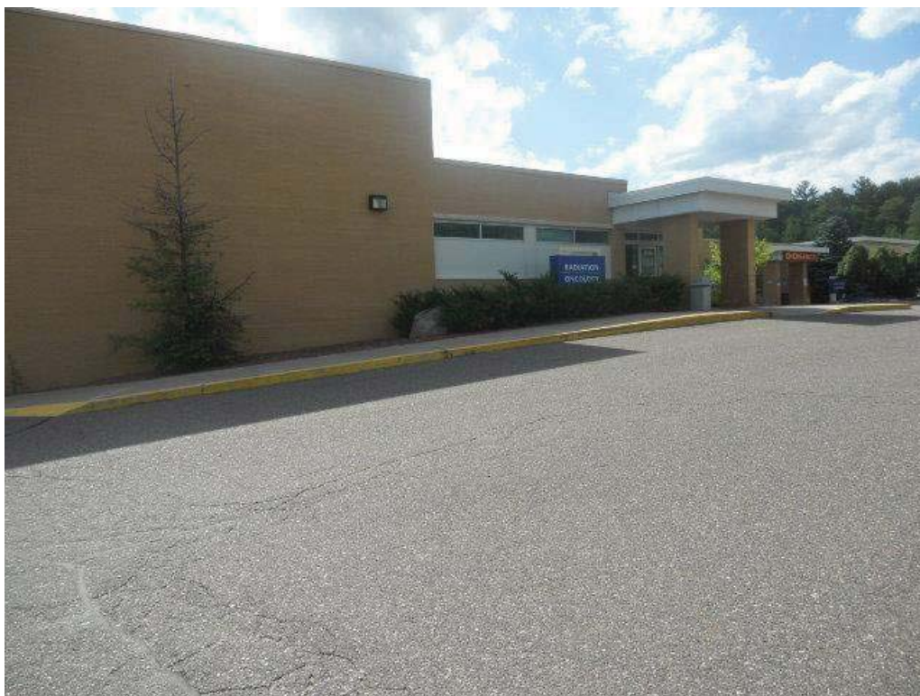
East Side of Building
