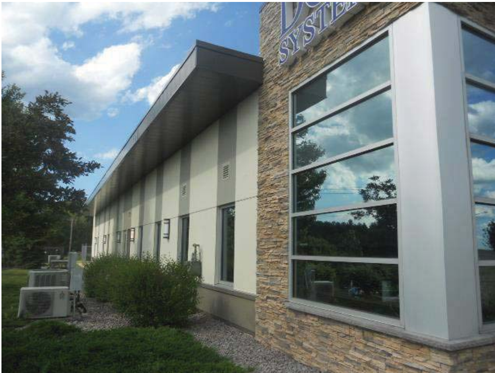
West Side of Building
