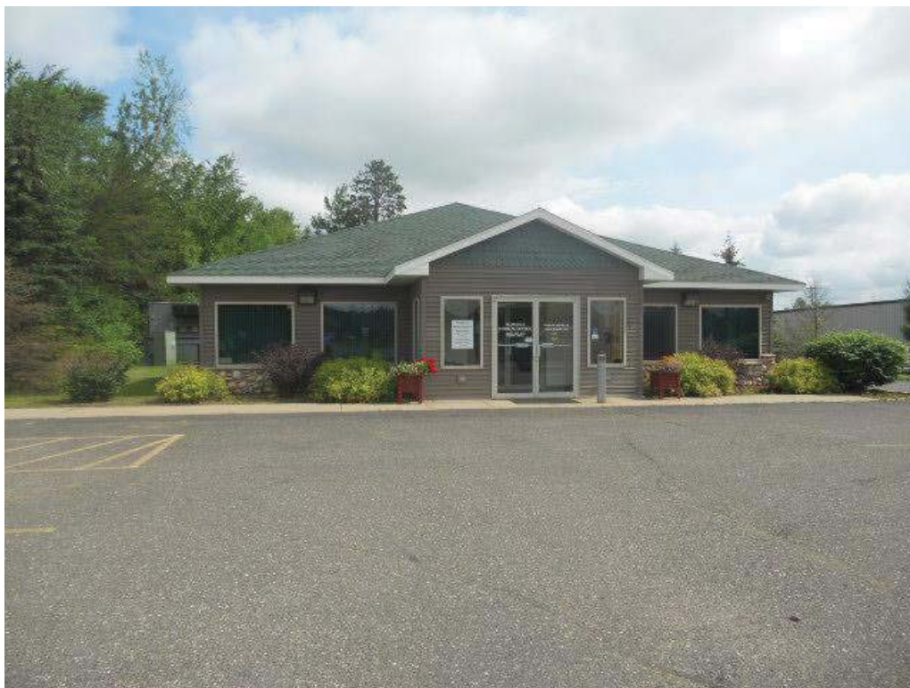
Front of Building
