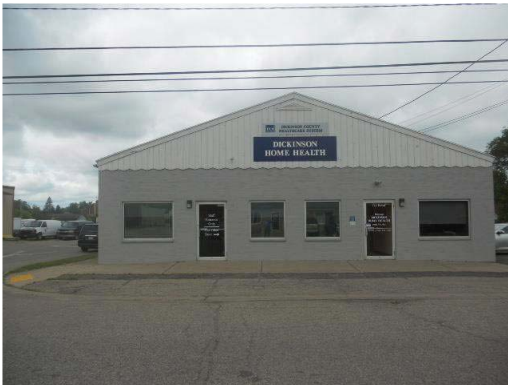
Front of Building
