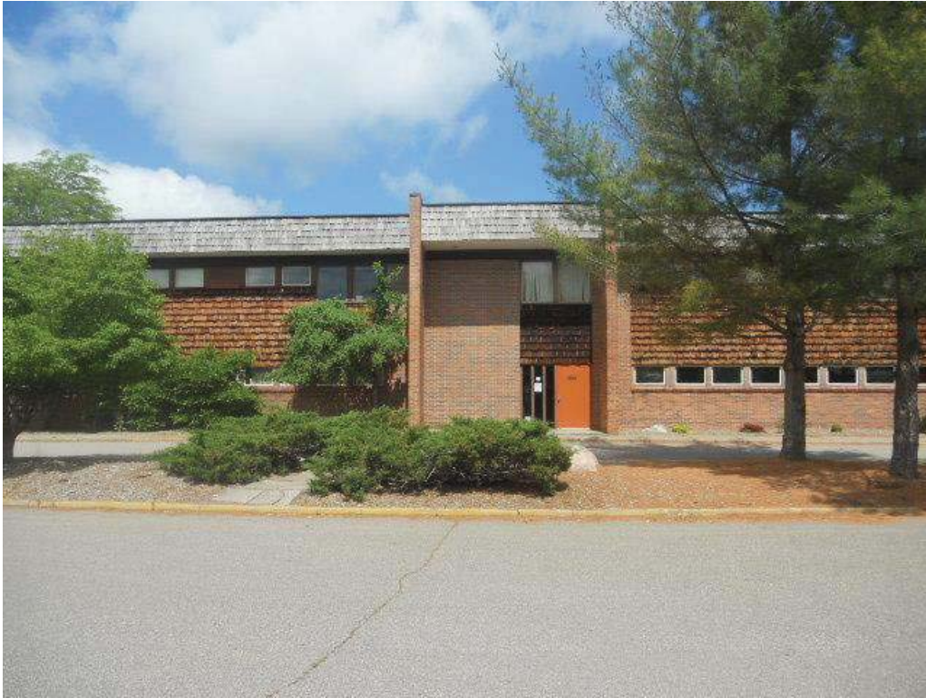
East Side of Building
