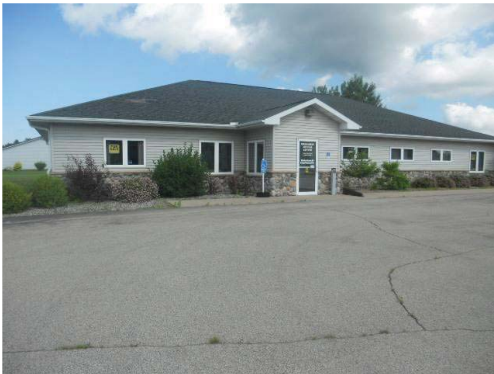
Front of Building
