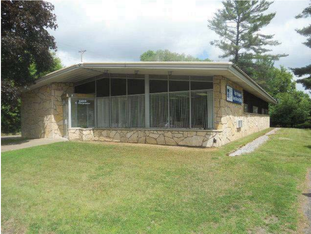
Front of Building
