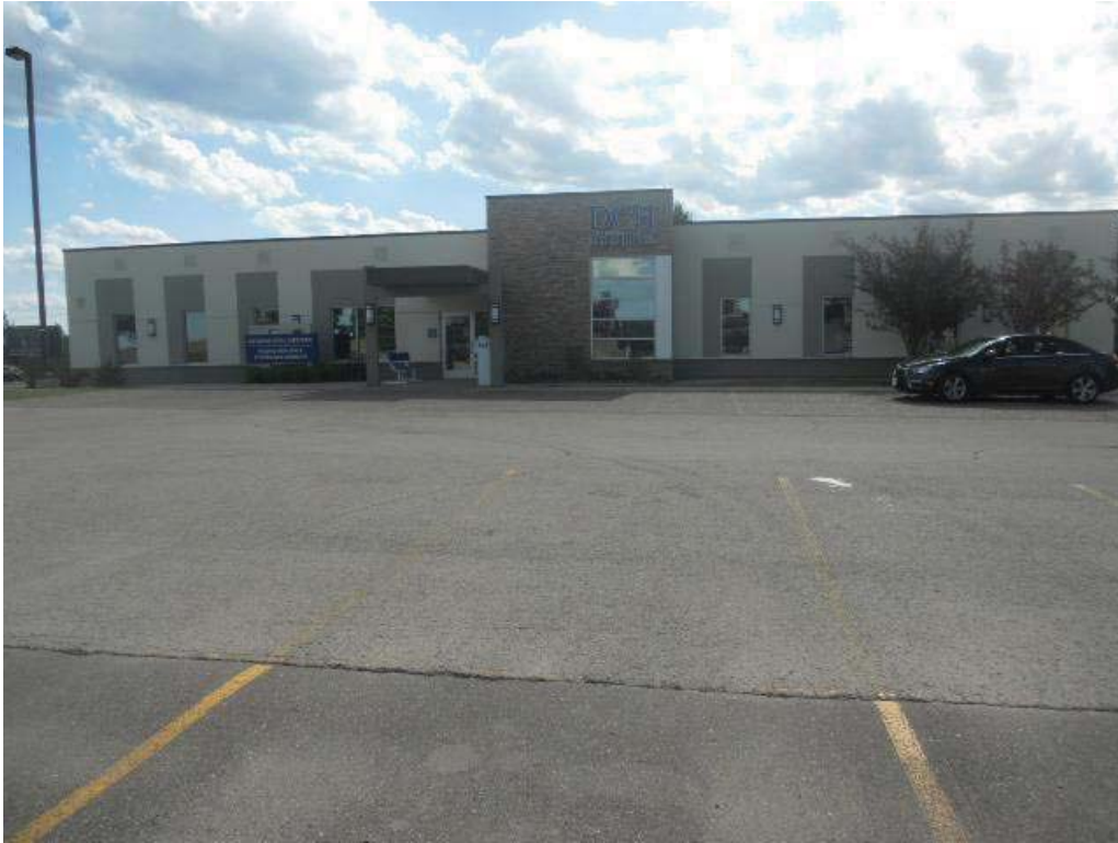
East Side of Building
