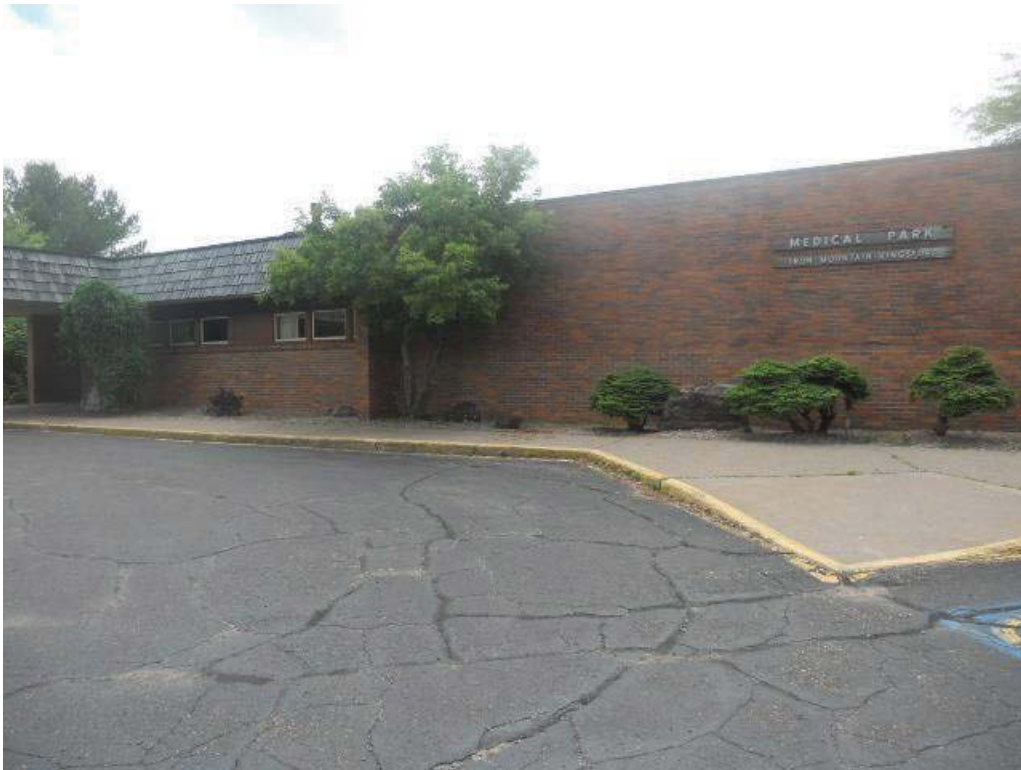
West Side of Building
