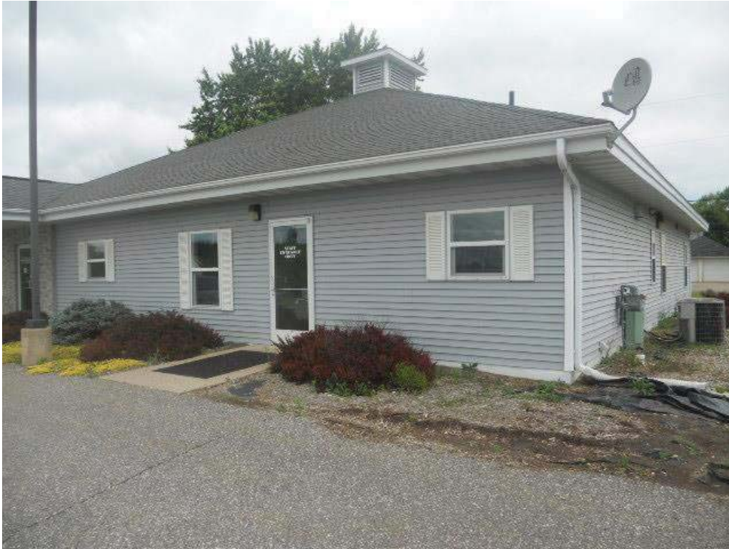
Front Side of Building
