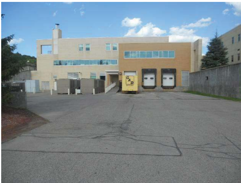
West Side of Building
