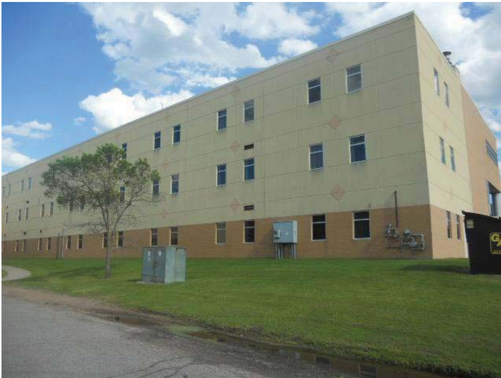
North Side of Building
